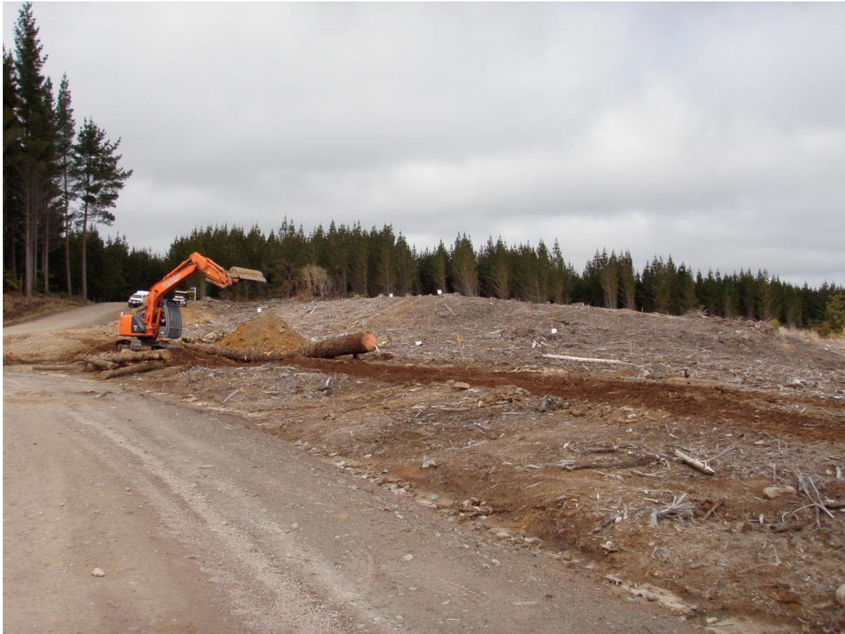
Figure 4: View of South East corner, note park road adjacent and horse trail between road and trial
