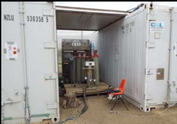
Vapormate set up.
