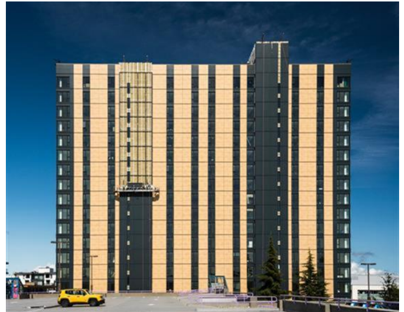
53 m tall timber building Vancouver, Canada
